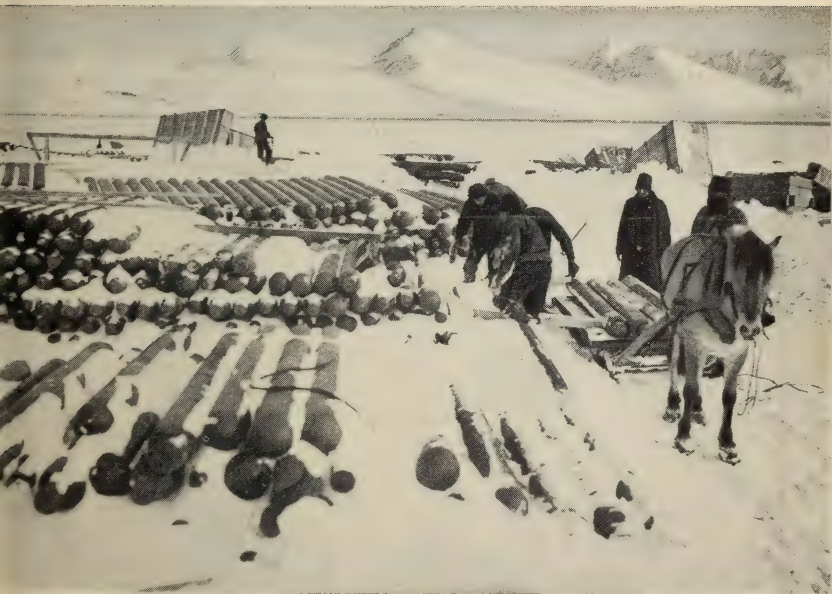
KING'S BAY—HAULING MATERIAL FOR THE MOORING-MAST. THE HYDROGEN TANKS.
